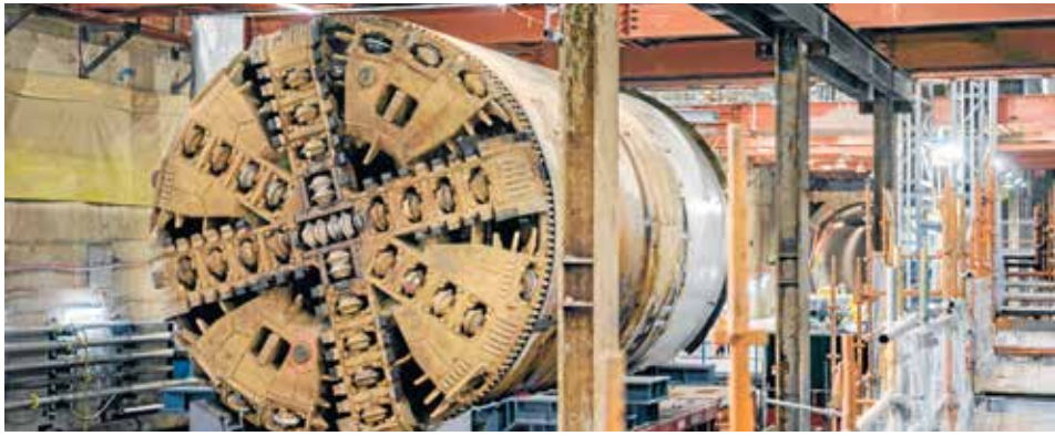
▲ TBM reassembly at Anzac Station – credit: The Metro Tunnel Project
